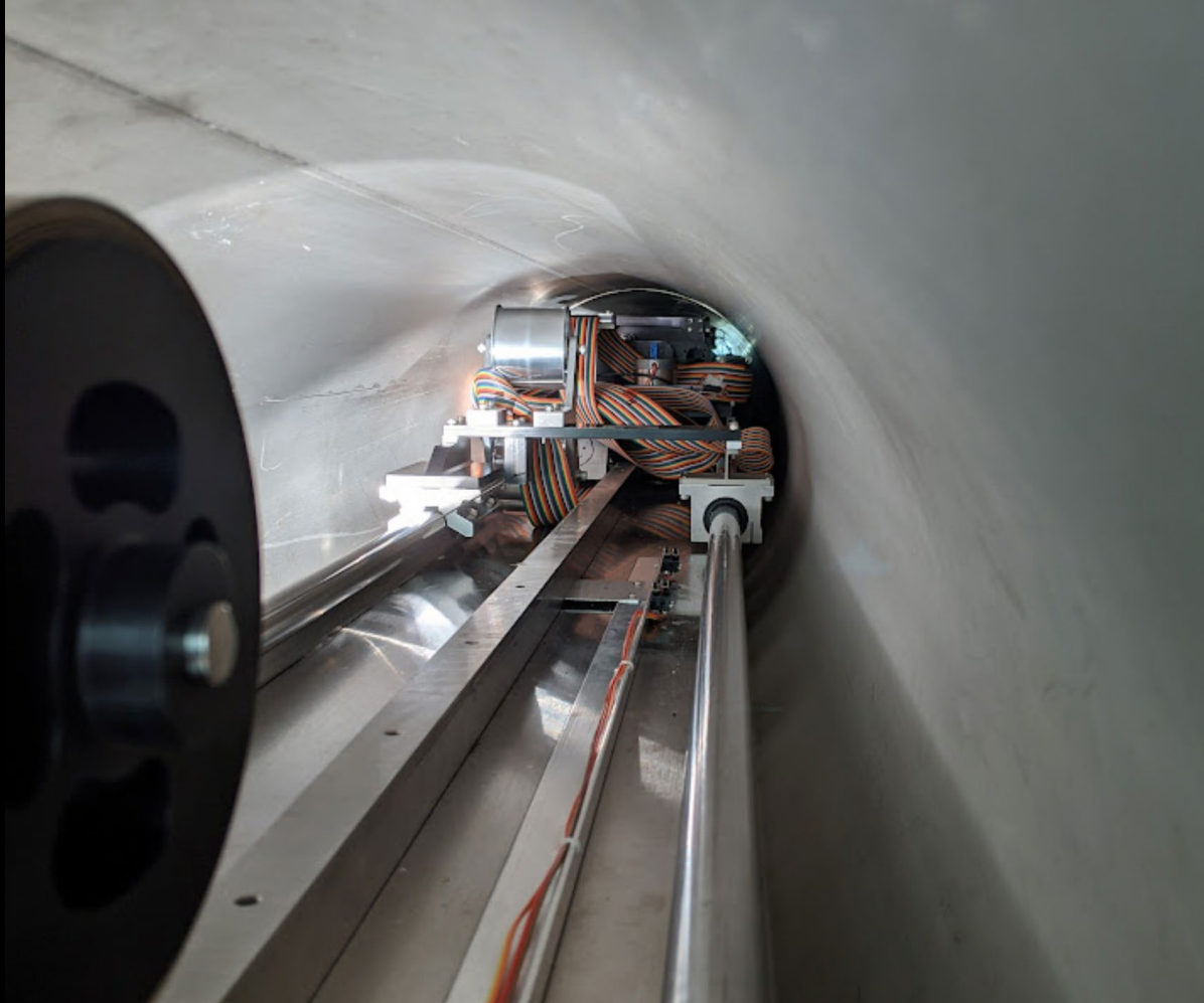
Image: Failure of Ribbon Cable System Inside FDL
